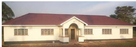
Newly built NCC admin block
